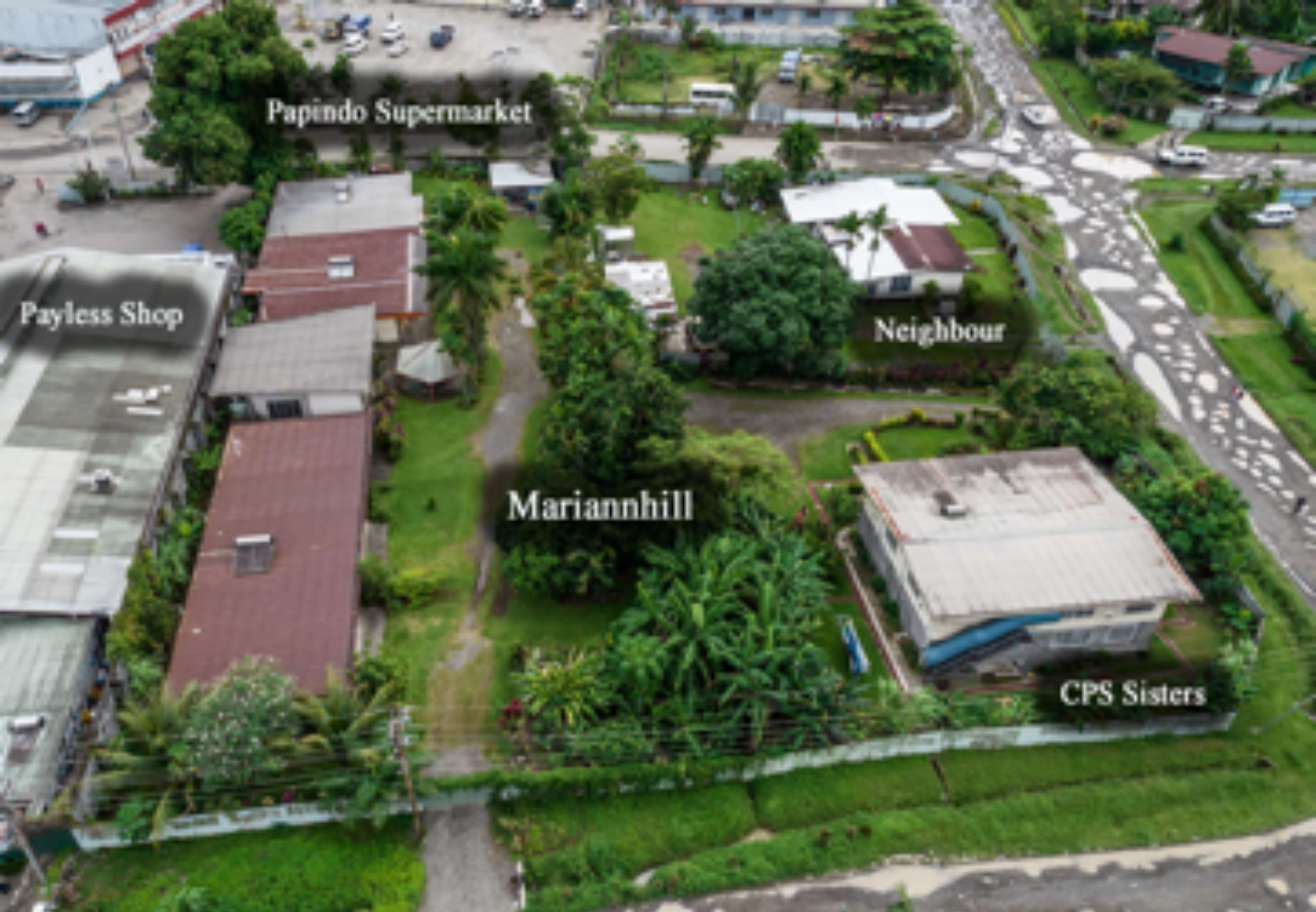
Drone Photo: Mariannahill House, CPS Convent in Eriku Lae
